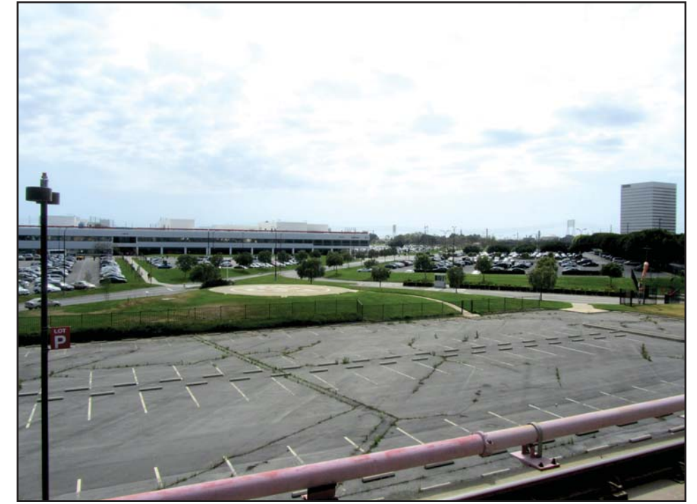
Existing onsite structures and parking from Metro Green Line platform.
